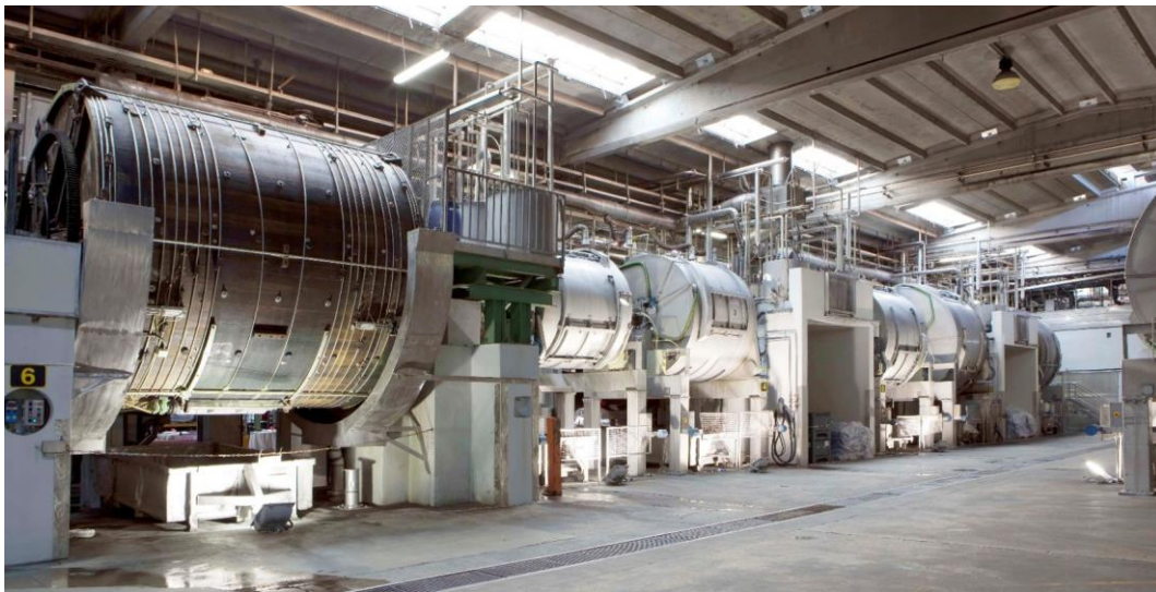
Fig. 2: Overview of one of the tanneries of the Gruppo Mastrotto in Arzignano, VI, Italy
