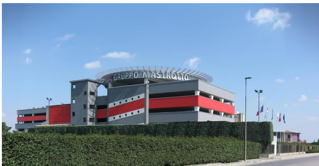
Fig. 1: Headquarter of the Gruppo Mastrotto in Arzignano, VI, Italy
